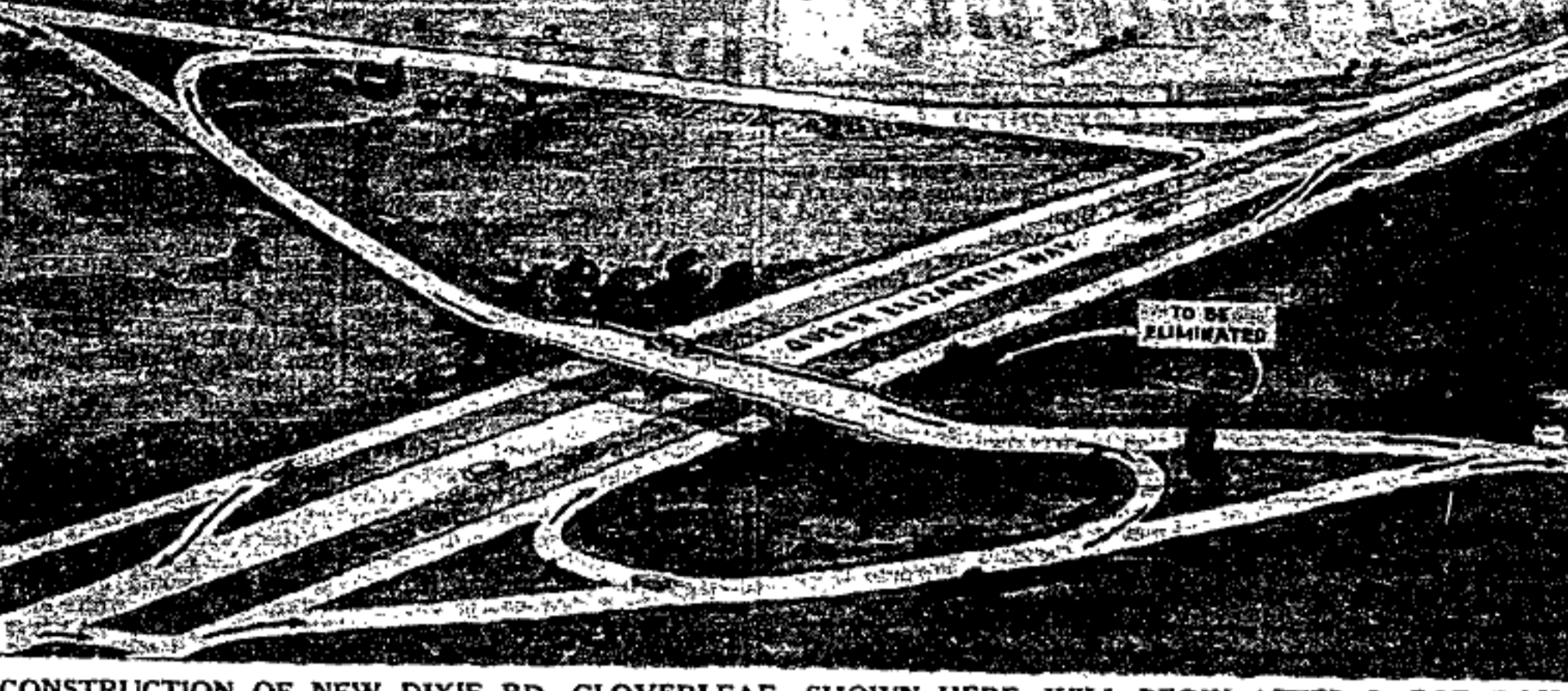
CONSTRUCTION OF NEW DIXIE RD. CLOVERLEAF, SHOWN HERE, WILL BEGIN AFTER LABOR DAY
